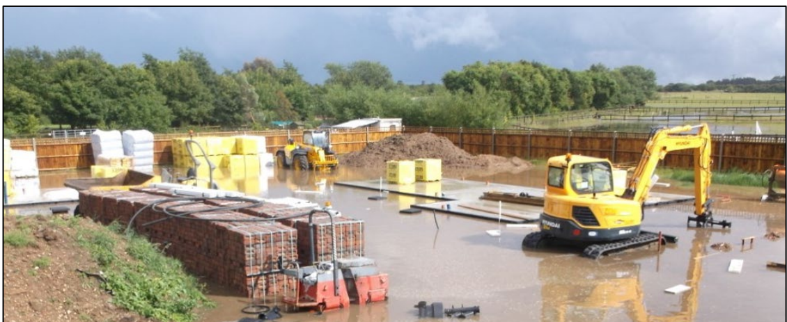
Photo 5: Photo of a development site located on the mapped surface water flood path that flooded in 2016, Hemsby, Norfolk.
