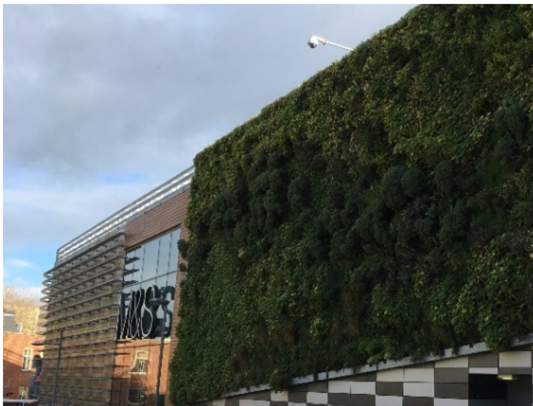
Photo 13: Photo of a green wall on a commercial building in an inner-city area, Norwich, Norfolk (Image E Simpson @ NCC LLFA)
