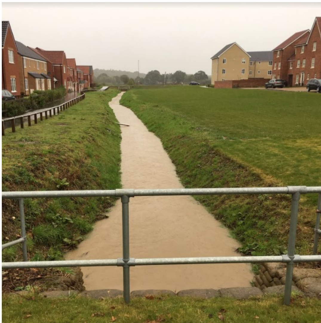
Photo 8 ordinary watercourse in North Norwich which is near bank-full during a rainfall event
