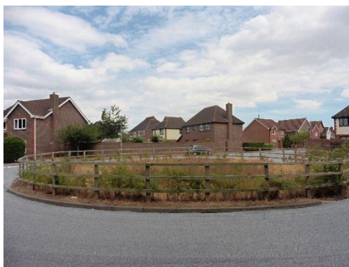
c) Badgers brook roundabout with dropped kerbs and storage created in the centre, overflow installed back to sewer system
