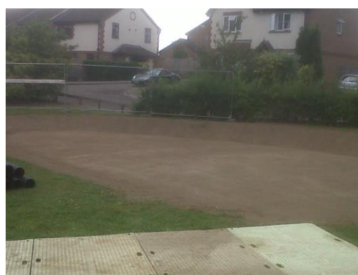
d) 2014 During construction – badgers brook roundabout and one of the shallow attenuation basins. The site flooded during construction and SuDS needed remedial action and additional community engagement to resolve concerns over the performance of the works. The parties, including the LLFA, learnt that any scheme may need construction plans and potential temporary measures during construction to prevent adverse impacts.
