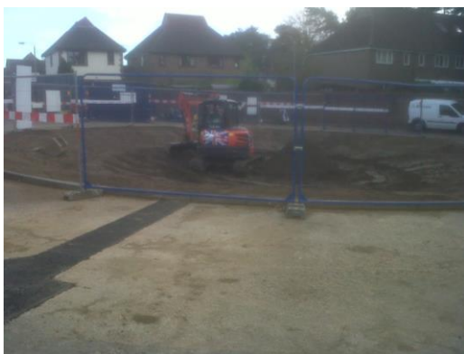
d) 2014 During construction – badgers brook roundabout and one of the shallow attenuation basins. The site flooded during construction and SuDS needed remedial action and additional community engagement to resolve concerns over the performance of the works. The parties, including the LLFA, learnt that any scheme may need construction plans and potential temporary measures during construction to prevent adverse impacts.
