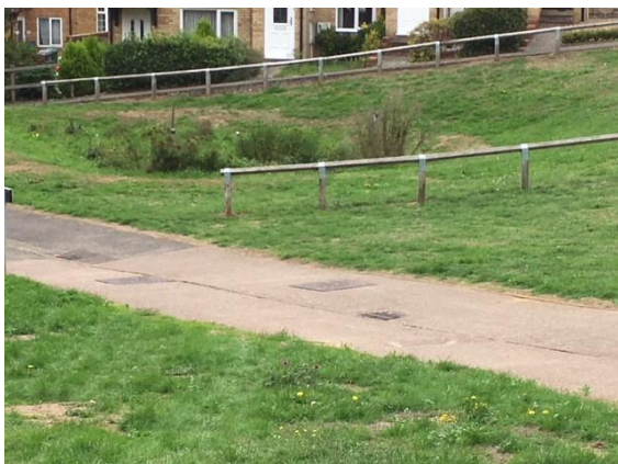
a) 2018 – raingarden with overflow back to sewer system
